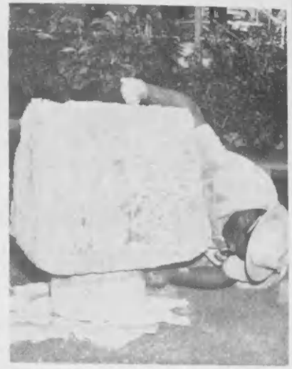
FINISHING TOUCHES complete the foundation holding masonry from one of Lago's original structures. The 1925 section is set in front of the Adm. Building.
